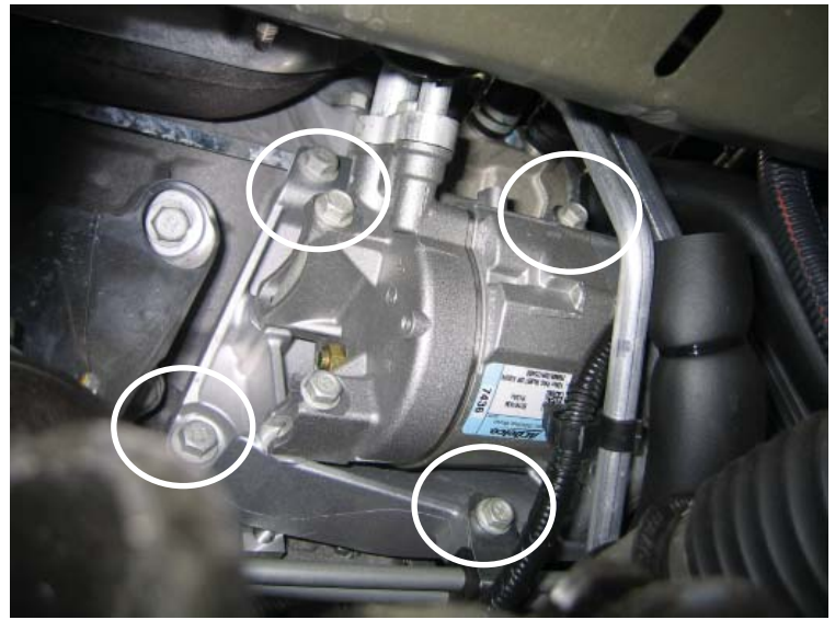
Remove (4) A/C Compressor Bolts
