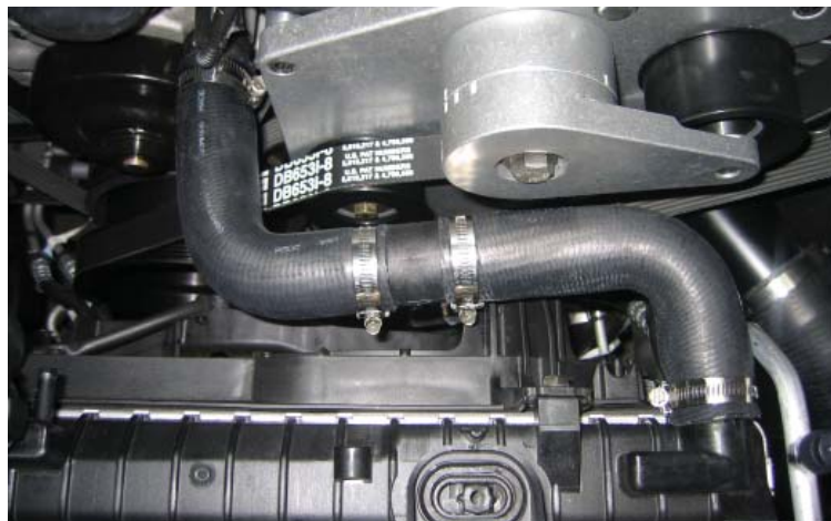
New Coolant Lines Installed
