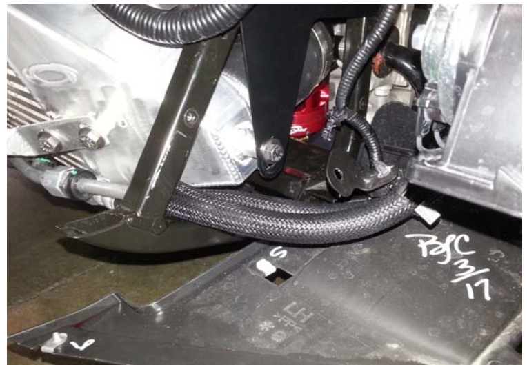
Transmission Cooler Lines
